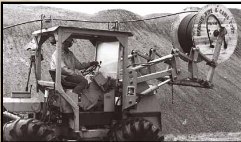
Lineman David Ripp assists in burying cable in 1987. Jackson Electric Cooperative now hires a contractor to install underground cable.
