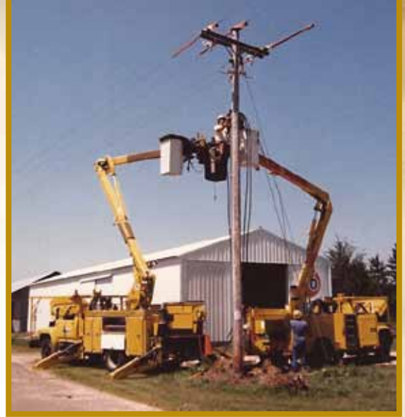
Linemen Bruce Hunter, David Ripp and Dan McKevitt work on a three-phase line in Millston near Deli, Inc.
