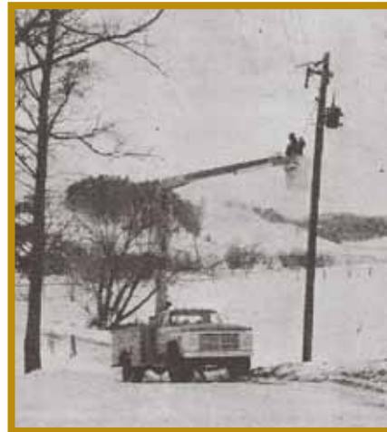
Lineman Arlan Danielson prepares to fuse a transformer for a member using the new basket truck. The new basket truck will replace one service truck and will be used to great advantage for changing transformers, breakers, insulators and also hot line work.
