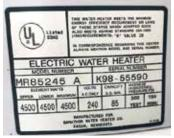
This is the sticker on the 85-gallon water heaters needed for warranty replacements. The 105 and 100-gallon water heater stickers are similar in appearance.
