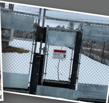
Above: Animal guards are installed on substation equipment to aid in the prevention of outages.
