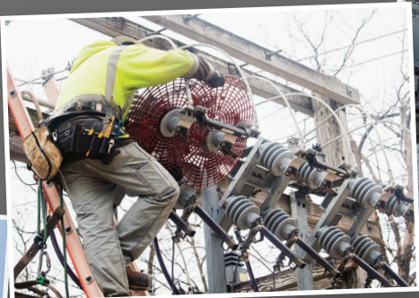
Above: Animal guards are installed on substation equipment to aid in the prevention of outages.
