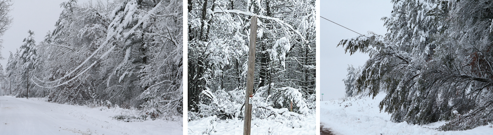
Left: The power lines were hanging low from the weight of the snow. Middle: Surprisingly, Jackson Electric wasn't challenged with many broken poles during the storm. This pole on County Road E wasn't so lucky. Line crews have already replaced this pole. Right: This tree came close to taking out this power line on County Road E.
